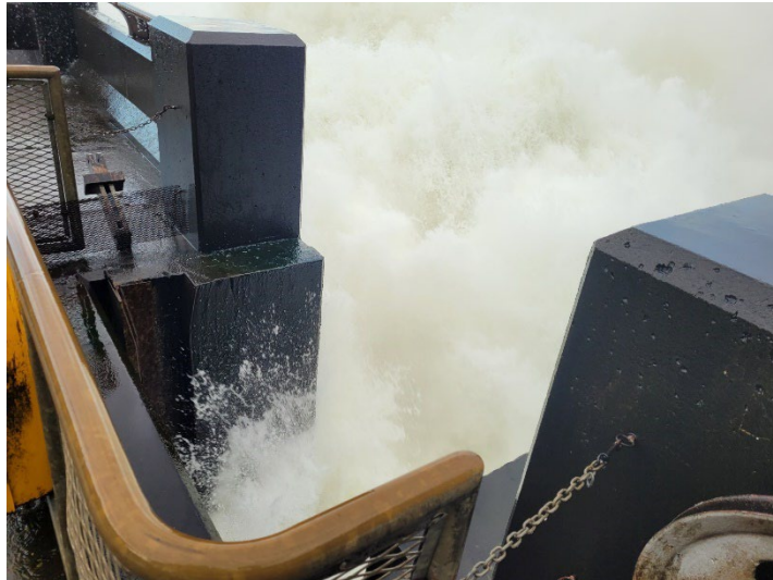
Figure 3: Location of old entrance weir within spillbay 20 discharge.
